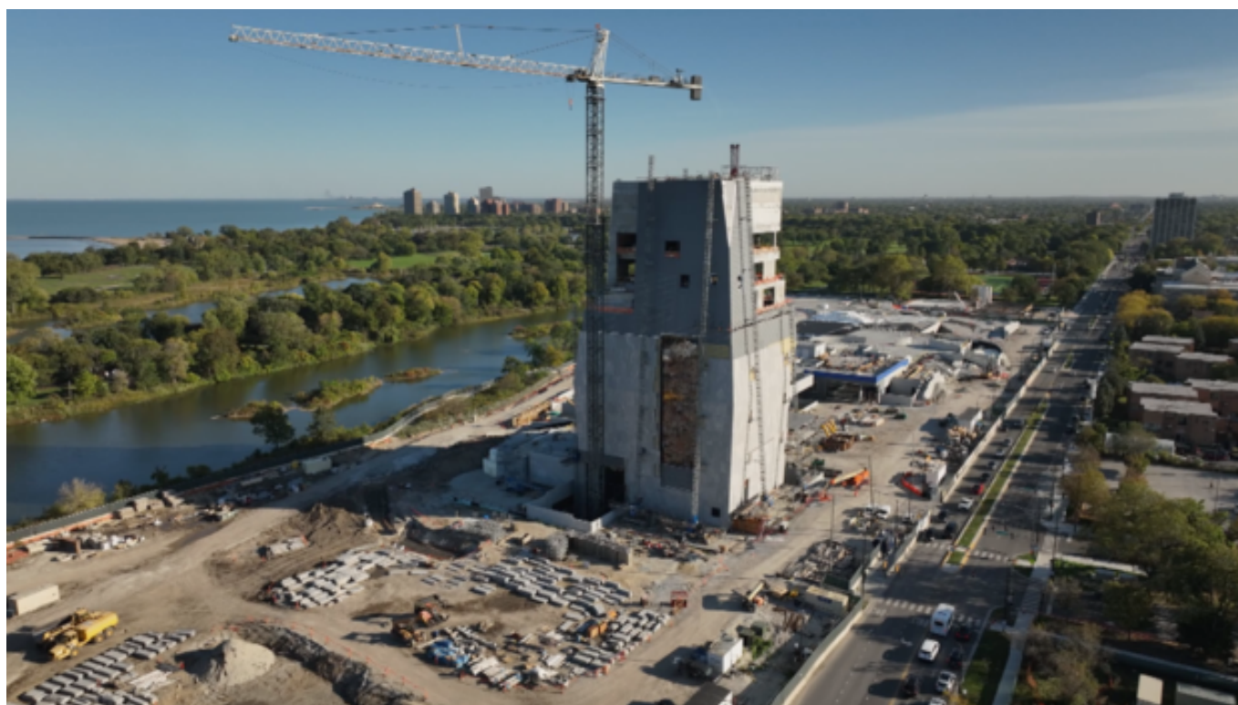
The Obama Presidential Center under construction in October 2024.
