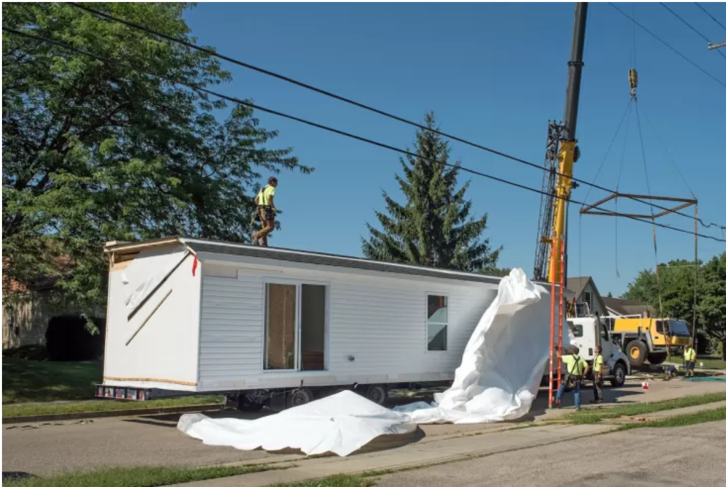
A modular home being installed. | lawcain / Adobe Stock
