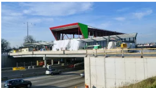
Eyes on the Street: 95th Street Station Work Is Rolling Along
