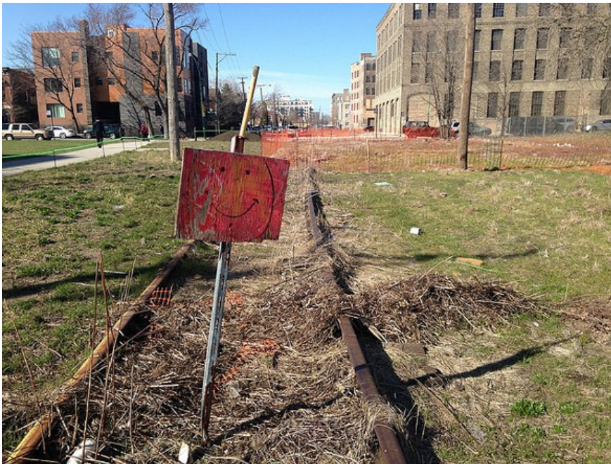
Abandoned BNSF rail line near 21st and Sangamon, which will become part of the Paseo this summer.
